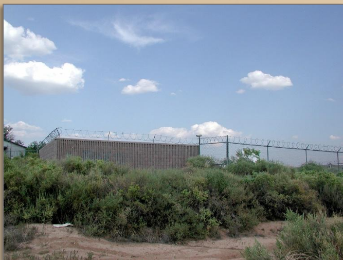
Sewer Pump Station
